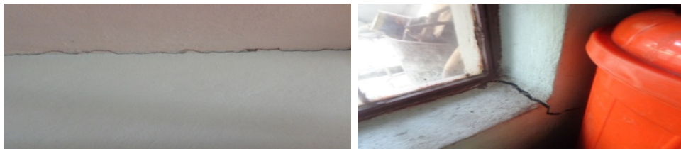
Figure 2(d): A crack line between the roof and the wall of the ground unit and upper floor Figure 2(e): Cracked Wall in one of the Units (both pictures show the same unit) (Pic. on the right)
