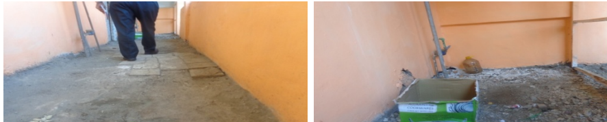
Figure 2(c): Dilapidated Corridor, Pipelines are Seen Exposed and Floor Tiles are Totally Removed
