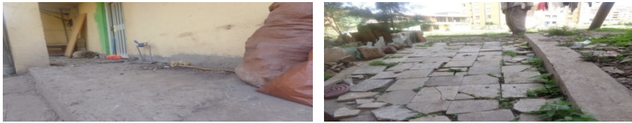
Figure 2(a): Dilapidated Corridor, Floor Tiles are Removed, Figure 2(b): The Removed Tiles are Used for Foot Path
