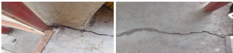
Figure 2(f): Cracks on Stair Case Joint between two Adjacent Condominium Blocks
