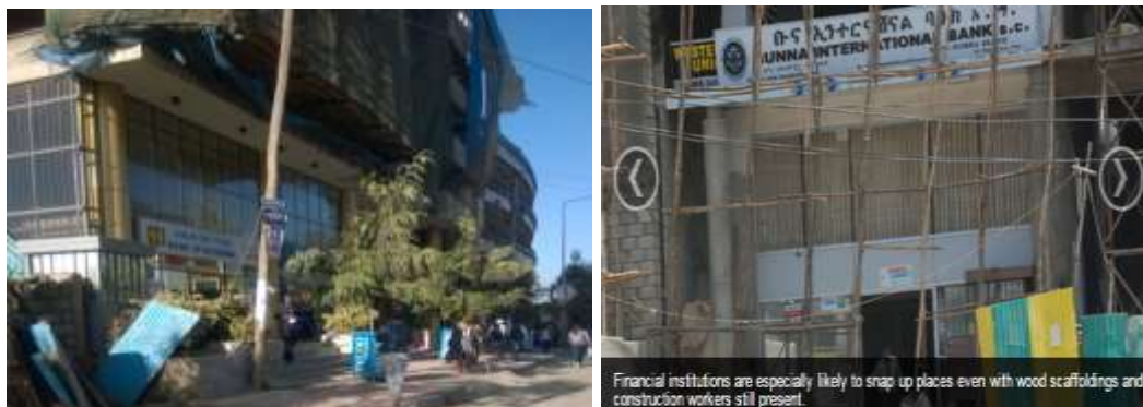
Figure 4.2 Rented Buildings under Construction
