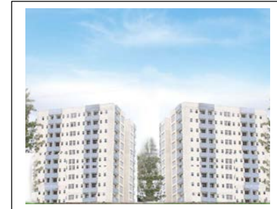
Employees Apartment G+10, 2 Buildings
